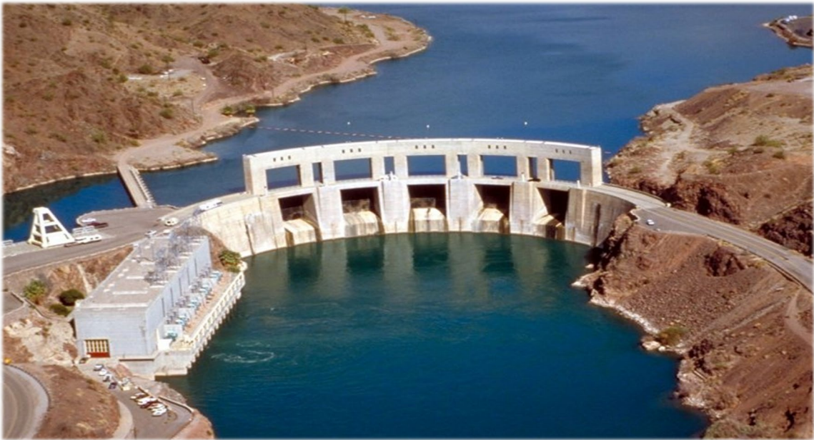
Figure 3.1: Parker Dam at Colorado River
