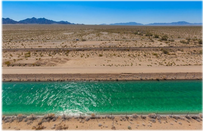
Figure 3.2: Colorado River Aqueduct
