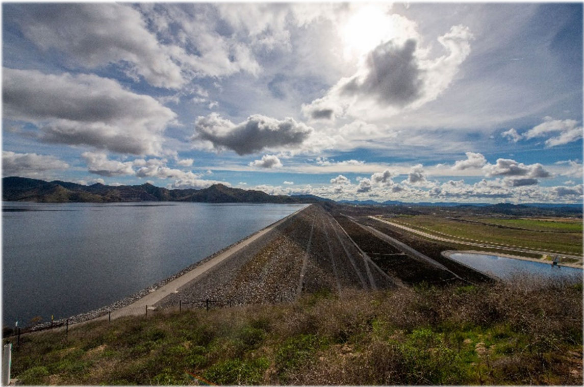
Figure 5.4: MWD’s Diamond Valley Lake (Potential Reserves for WSAP Allocations)
