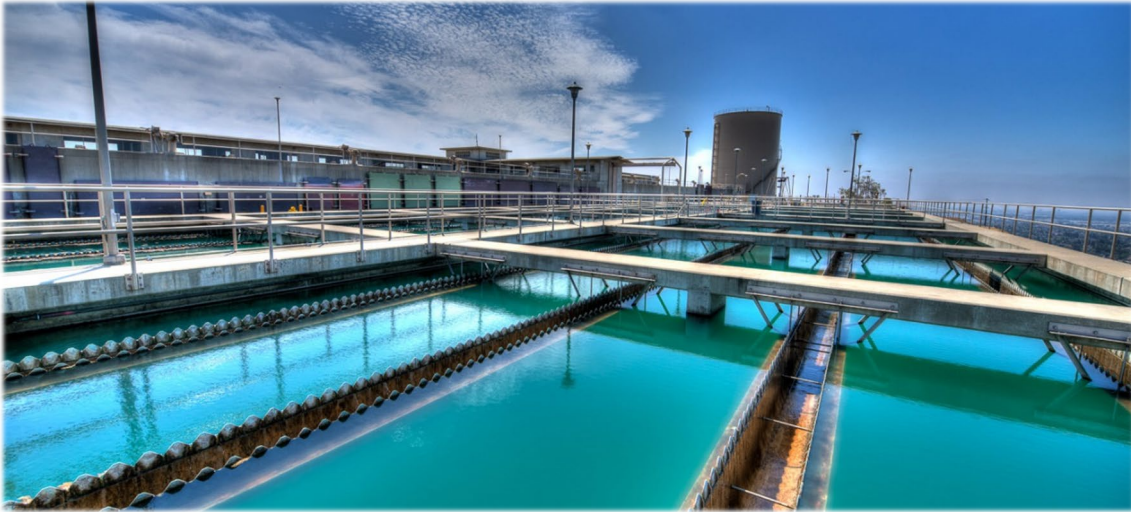
Figure 3.14: MWD’s Weymouth Treatment Plant Provides a Safe Supply of Water
