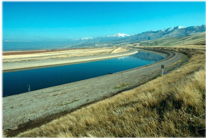
Figure 3.3: California Aqueduct or "SWP"
